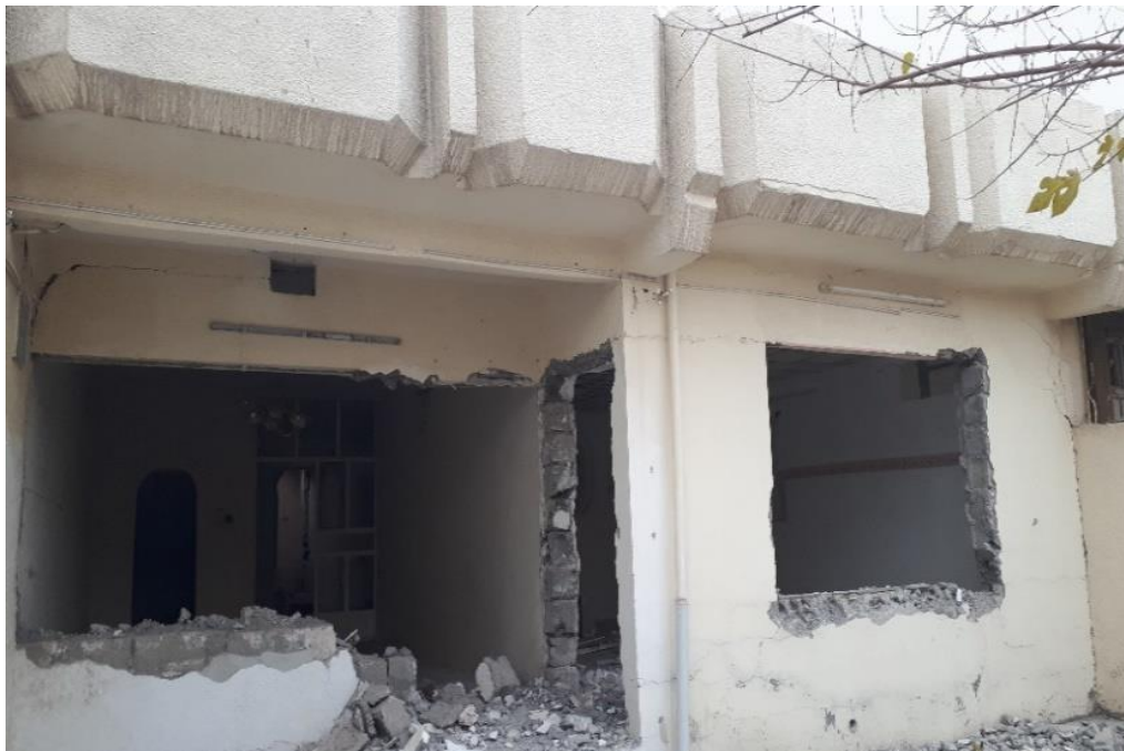
Figure 2. Old demolished house where the CDW was taken.
