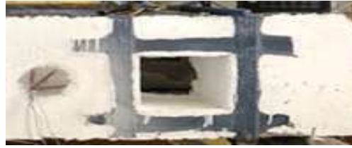
Figure 8. Application of Carbon Fiber Reinforced on opening .
