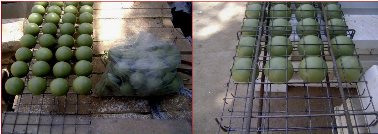
Figure 7. Preparation of Bubbled Slab Reinforcement.
