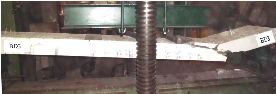
Figure 26. Crack Patterns and Failure Mode of Solid Slab (BD3).
