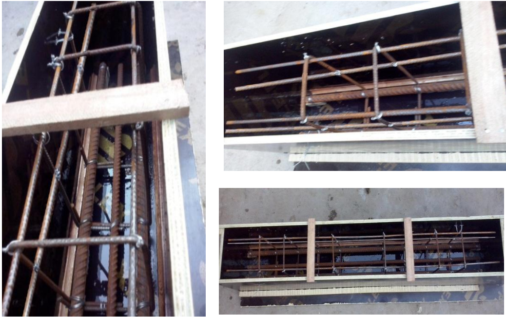
Figure 3. Mold fabrication and reinforcement cage of a typical tested beam.
