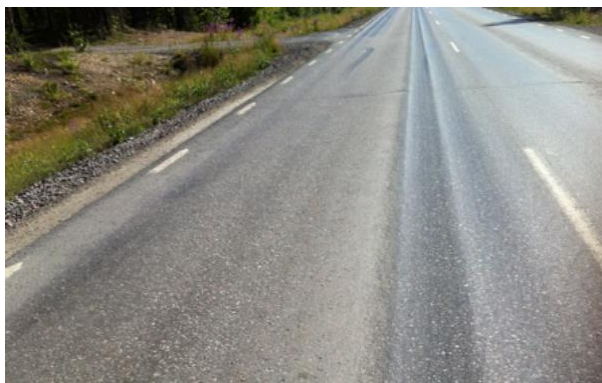
Figure 3. Cracking : the fracture that grows perpendicular to the pavement's axis.
