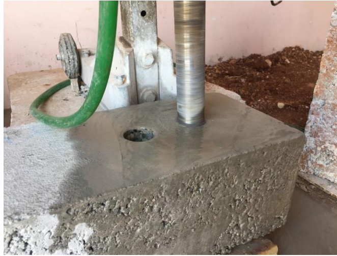
Figure 4. The coring cutting machine.
