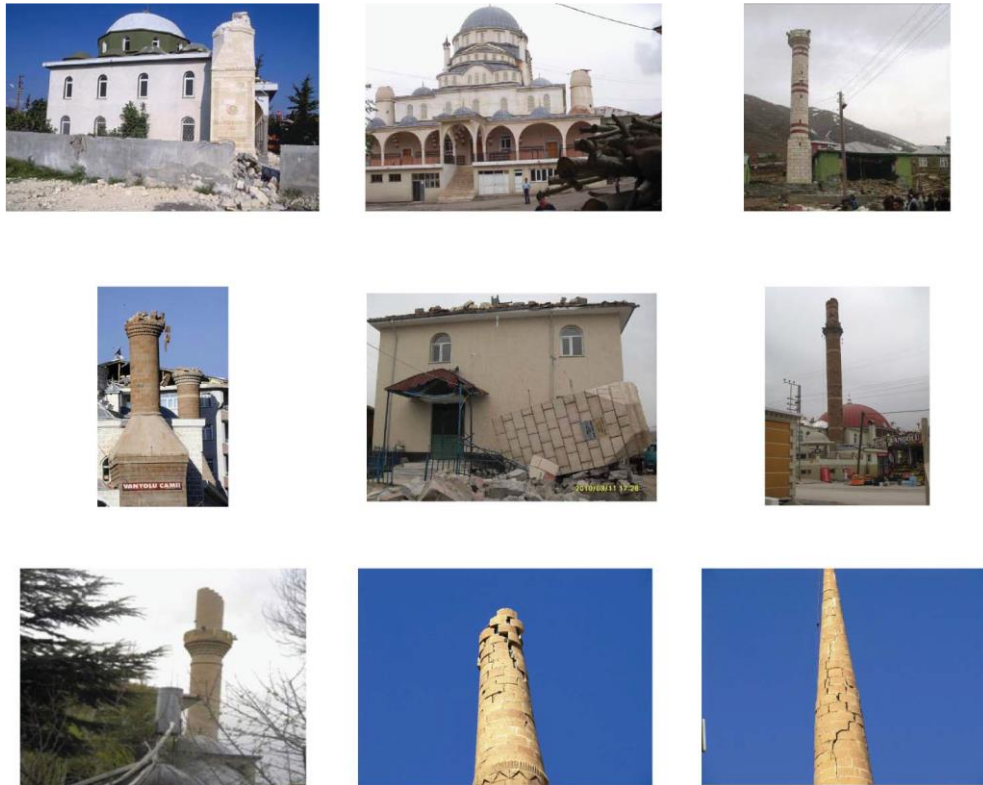
Figure 1. Collapsed masonry minarets (Mammadov, 2013)
