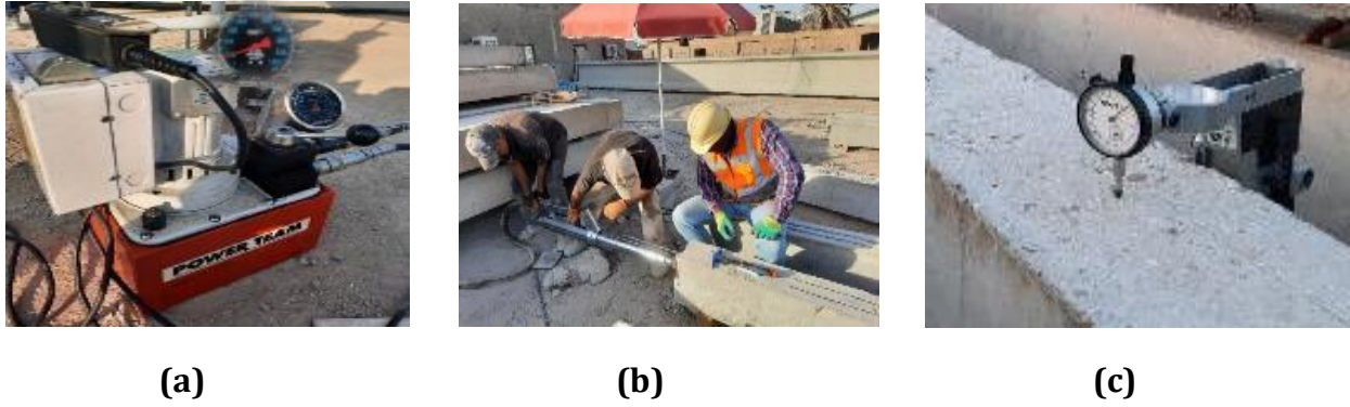
Figure 8. Operation of post-tensioning, a-PS equipment; b- PS process; c- camber recording
