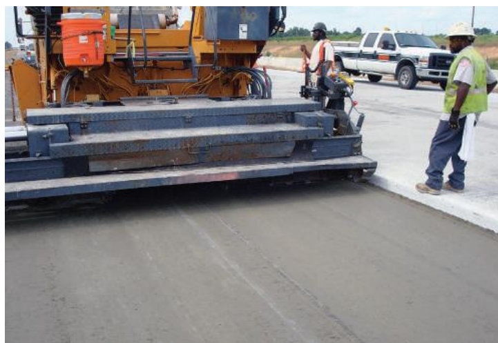
Figure 2. Setting up the RCC (Harrington et al., 2010).
