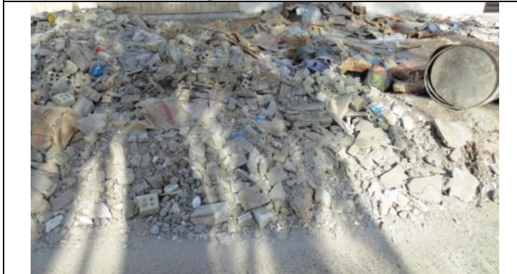
Excavation works & rubbles
