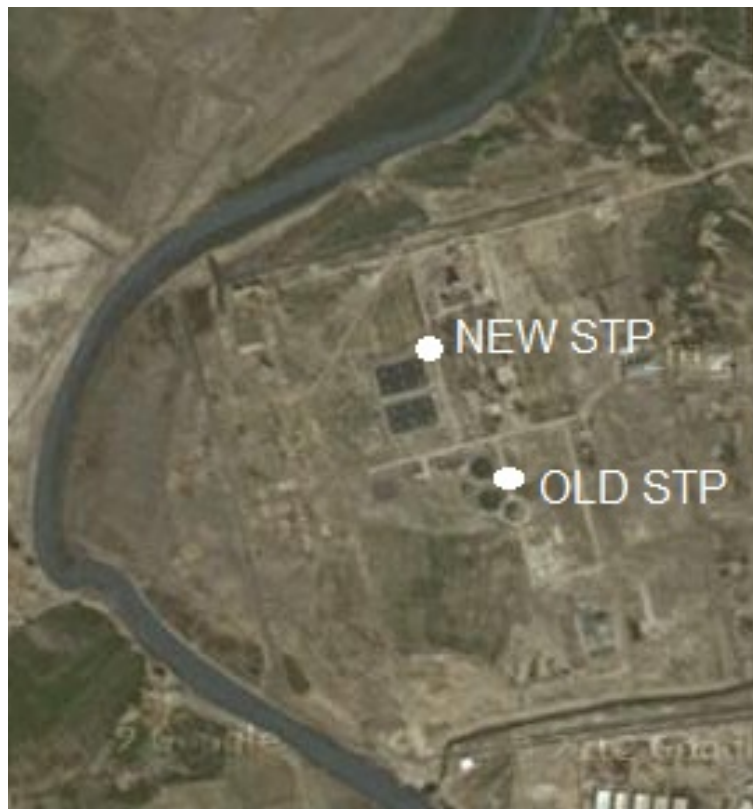
Figure 1. Google earth photo for Al-Diwaniya STP, Diwaniya project, Iraq.
