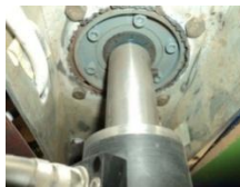
Figure 11. Connection between M420 rotary torque transducers and gearbox.
