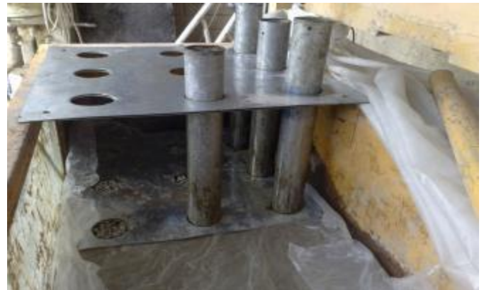
Plate 7. The process of stone column installation.
