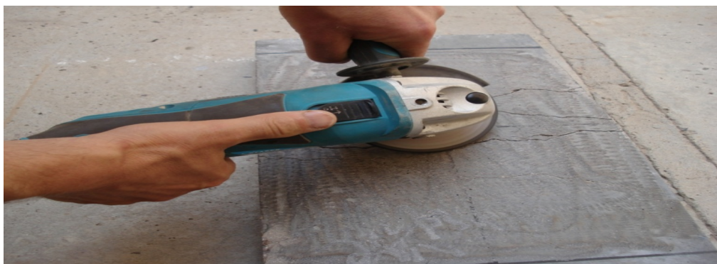
Figure 4: Concrete surface preparation by grinding
