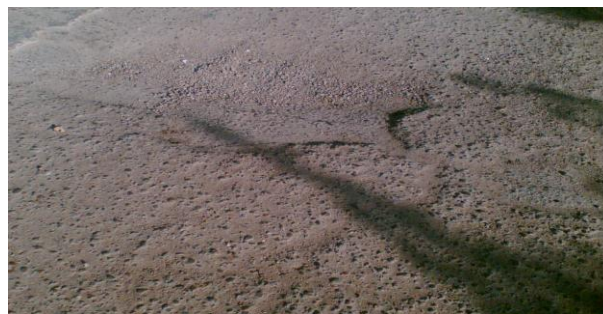
Fig (7) Patching at AL-Adel City
