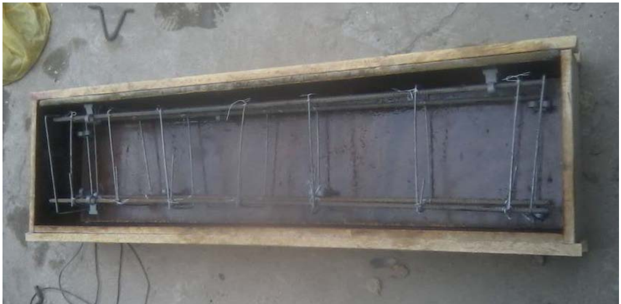
Fig.(1) Typical Moulds of Reinforced Concrete Deep Beams.
