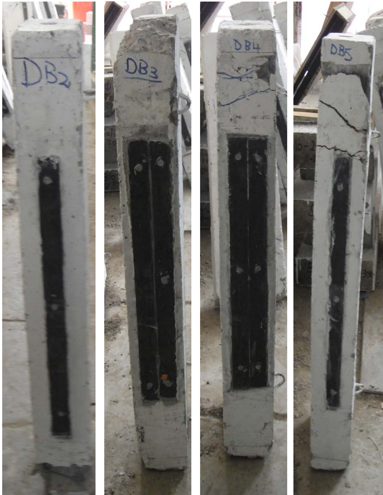
Fig.(6) Crack Pattern of Experimental Tested Retrofit Beams under Two Points Concentrated Load (at Tension Zone).
