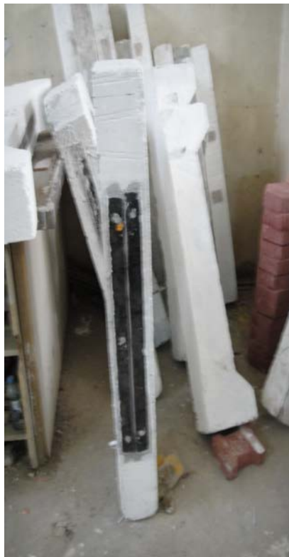
Retrofit Double Strips CFRP (DB3, DB4)
