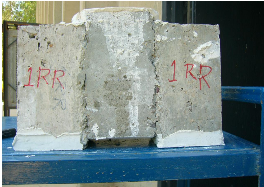
Fig. 6: Failure of Reinforced Specimen with Roughened Interface Surfaces to 6mm Amplitude.
