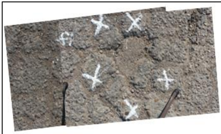
Figure 3. Ground control point around distress area.
