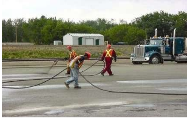
Figure 9. RCC Application of curing mixture (McLeod and Laughlin, 2001).
