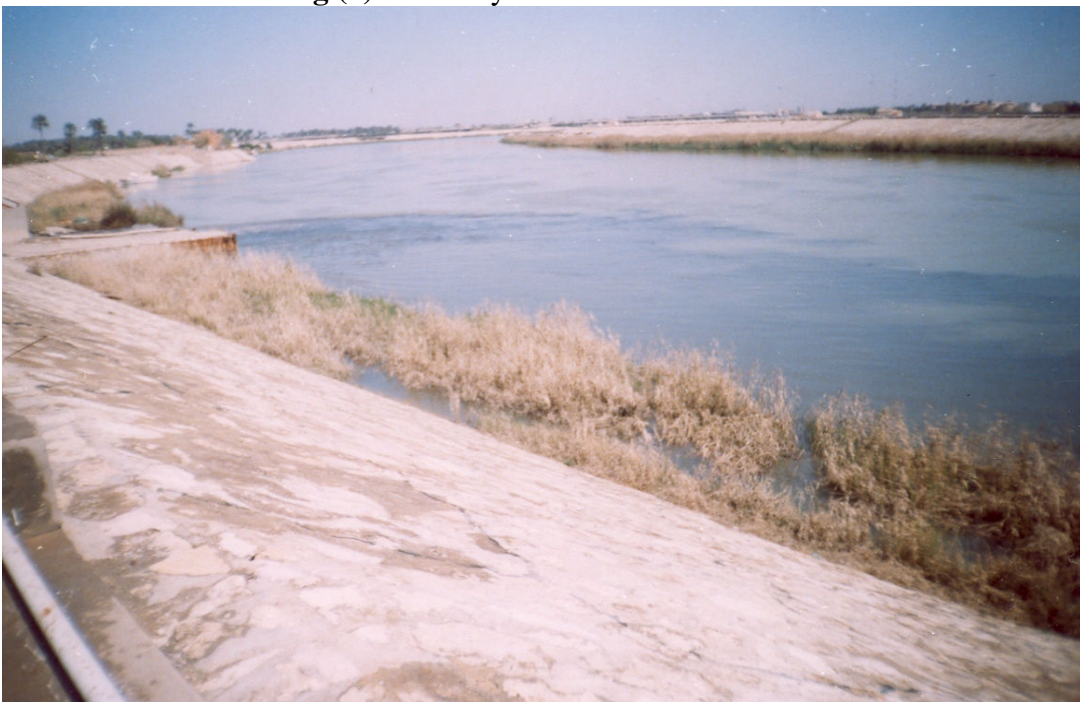
Fig (4) Raw sewage training along the river bank.
