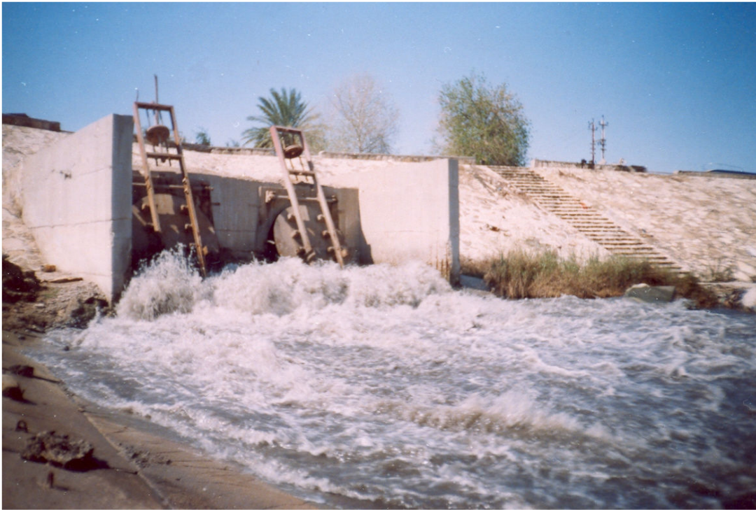
Fig (3) Al-Saidiya PN outfall structure.
