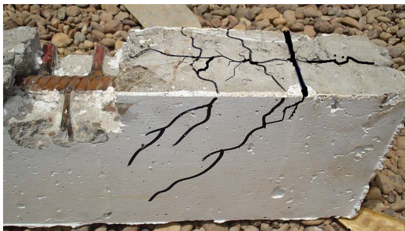
Figure (5): Crack pattern of beam B3 after failure
