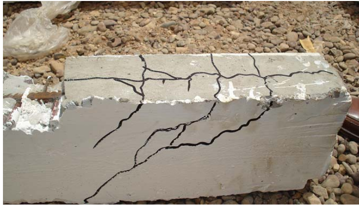
Figure (4): Crack patterns for beam specimen B6 with compressive strength 53MPa
