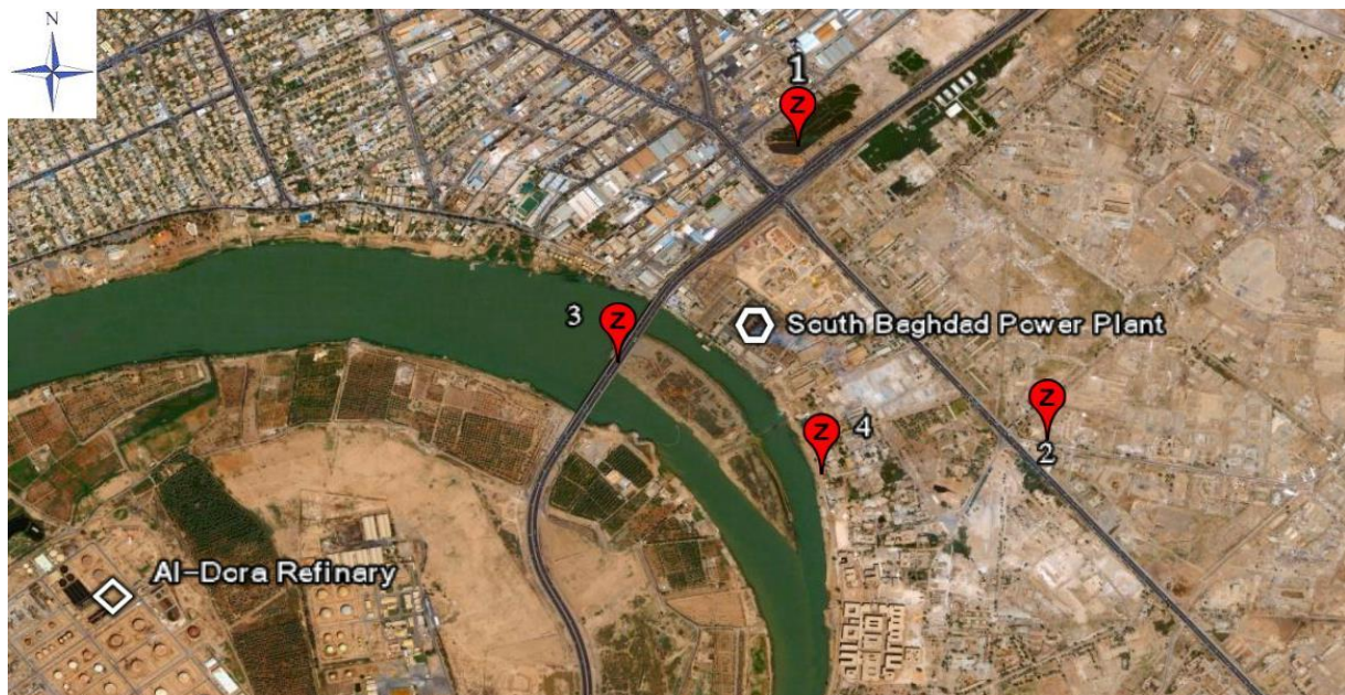
Fig.(5): Aerial photo for Al-Za'afarania area shows the measuring sits around the power plant.
