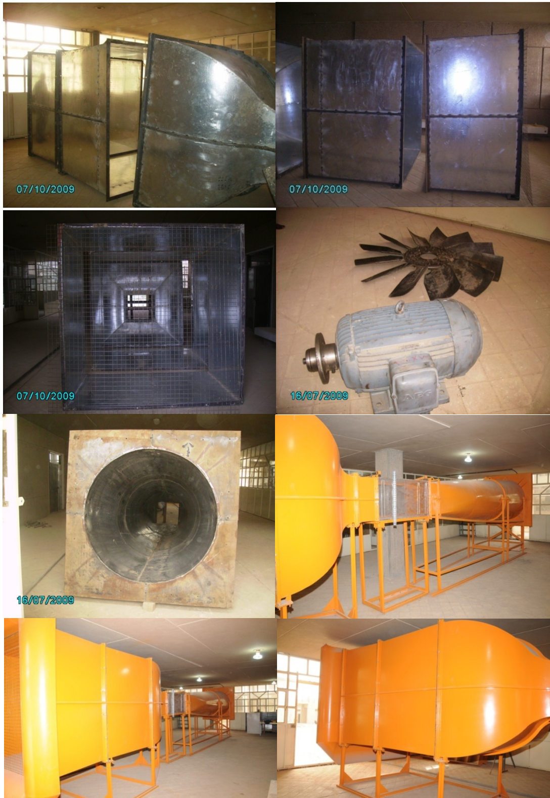
Fig.4: Wind Tunnel Construction.
