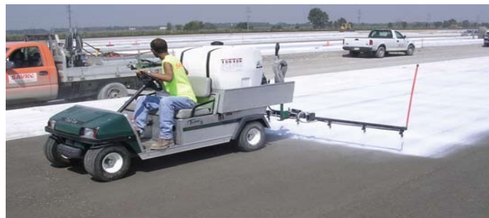
Figure 7. Application of curing compound (Dale et al., 2010)
