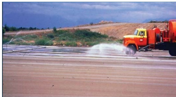
Figure 6. Moisture curing using sprinklers and fog spraying (Dale et al., 2010) .
