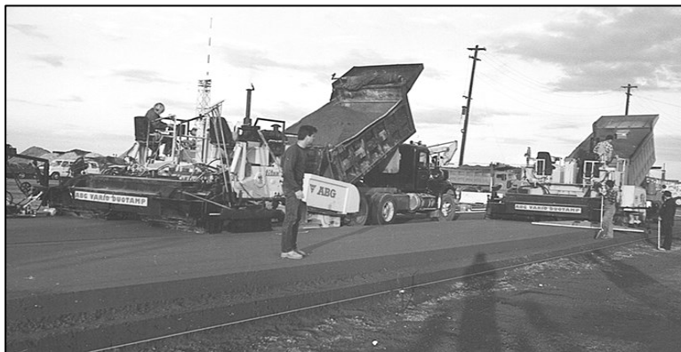
Figure 1. RCC placement using modified asphalt pavers (ACI 325.10R, 1995)
