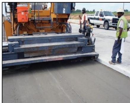
Figure 2. Paving the RCC ( Dale et al., 2010 )
