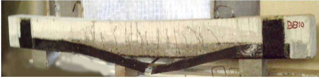
Figure 11 Crack pattern for beam BB10- strengthened beam (at bottom and side face by CFRP sheets)
