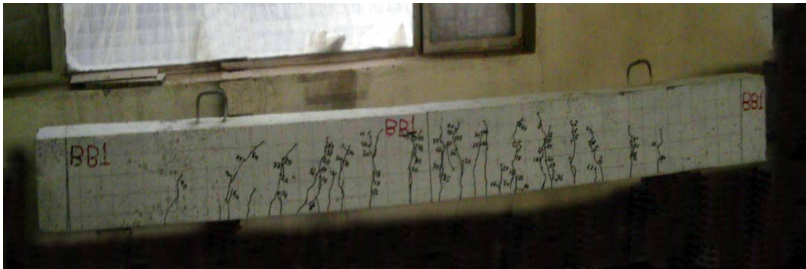
Figure 6 Crack pattern for beam BB1- control beam
