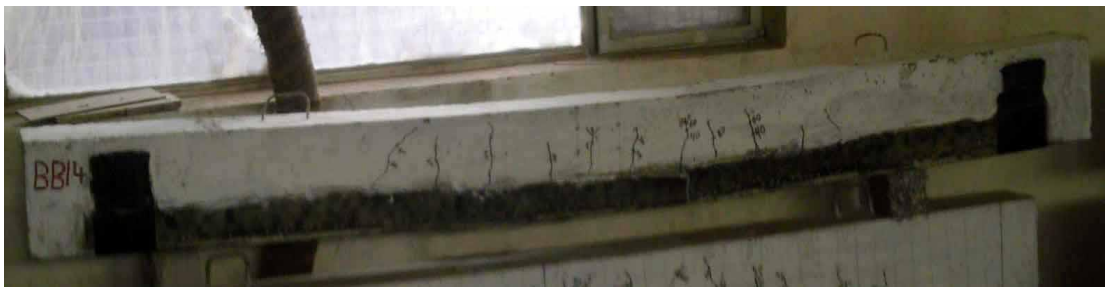
Figure 20 Crack pattern for beam BB14- (beam repaired by CFRP in side faces)
