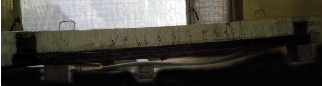
Figure 18 Crack pattern for beam BB13- (beam repaired by CFRP in bottom and sides)
