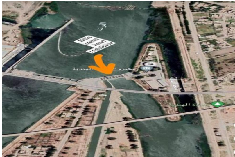
Figure 1. Hilla Canal Main Regulator (Google Earth).
