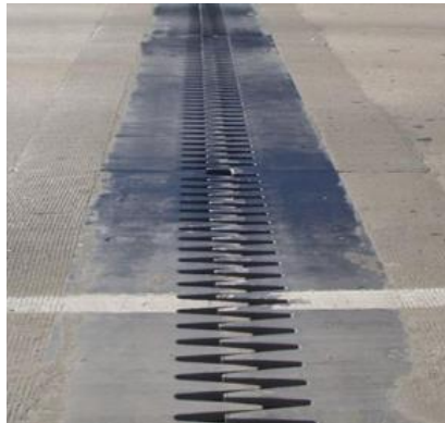
Figure 6. An Installed Armored Joint (Scansem Materials, 2024)
