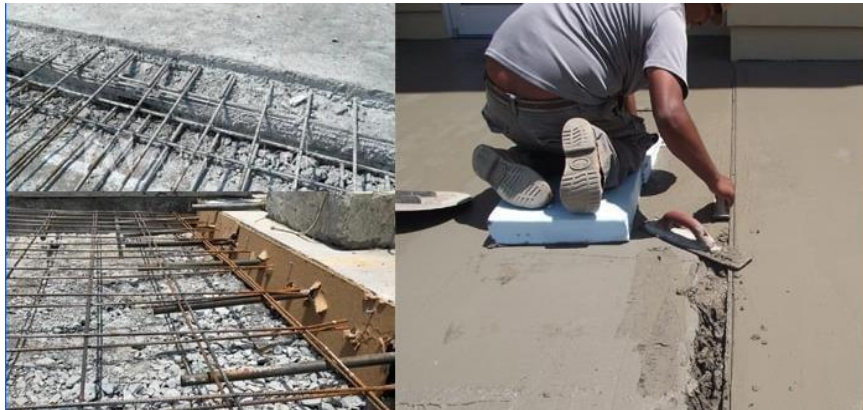
Figure 4. Example of construction joints (Steffen, 2023)
