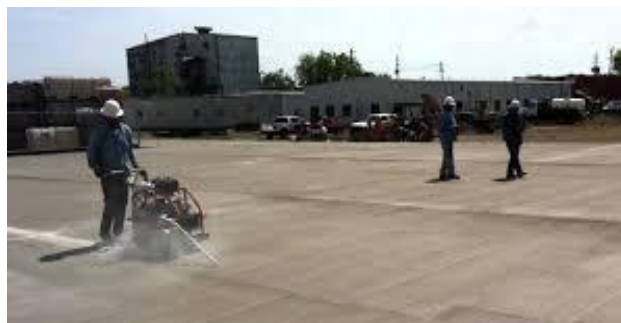
Figure 7. Saw-Cut Joints at the construction site (Rahman, 2024)
