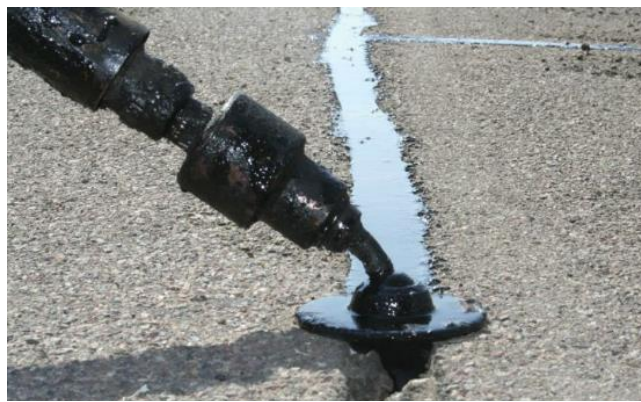
Figure 9. Process of applying joint-sealers (Woods, 2020)
