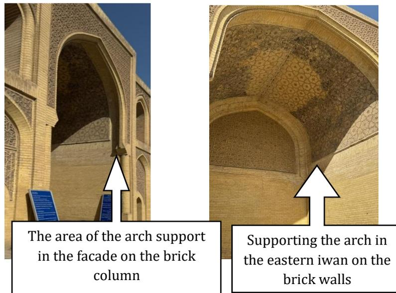
**Figure 12.** The Joints Between the Structural Elements that make up the Iwans, where the Brick Walls support the Largest Part of the Arch.
