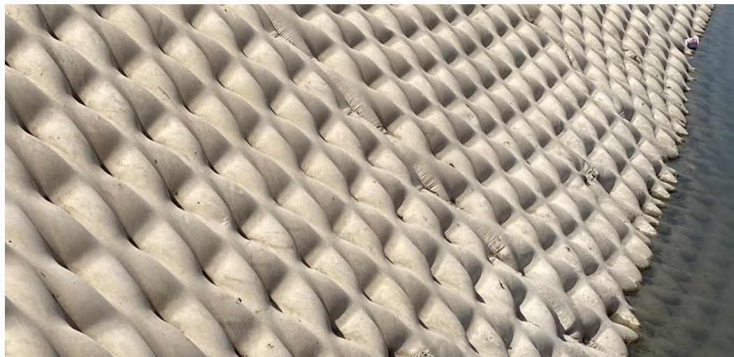
Figure 3. Image of concrete quilt lining of Bani Hassan Canal.
