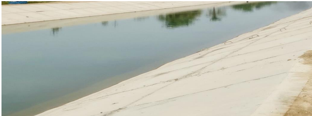
Figure 2. Image of the concrete lining of Bani Hassan Canal.
