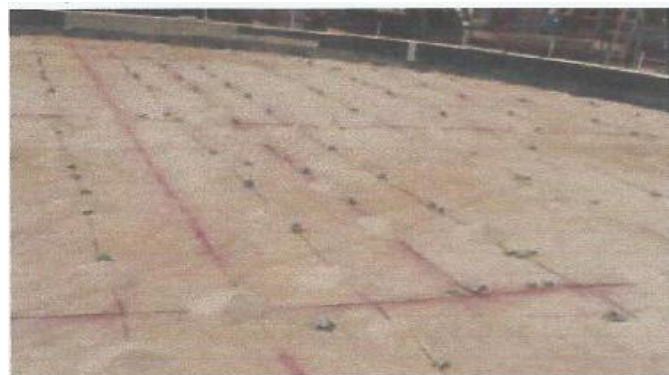
(f) ICCP grid anode system
