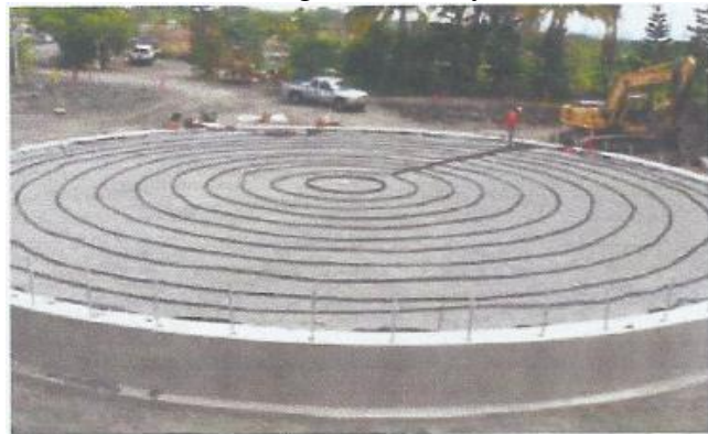
(g) ICCP loop anode system
