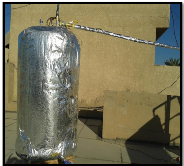
Figure 4-b. Water storage tank
