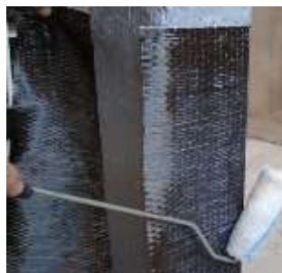
E- Wrapping the CFRP fabric sheet using a roller
