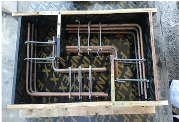
Figure 3. Typical mold with reinforcement.
