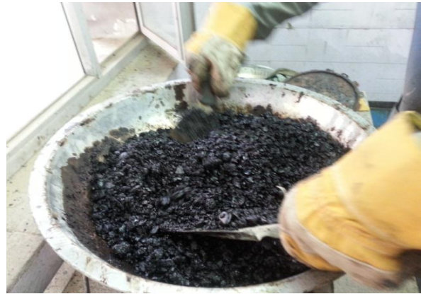
Figure 4. Mixing of Asphalt Mixtures.
