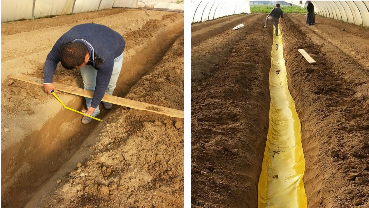
Figure 2. The installation process of the polyethylene sheet below the soil surface.
