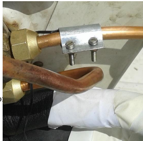
Figure 3. Photo of NTC thermistor and fixing it on tube surface.
