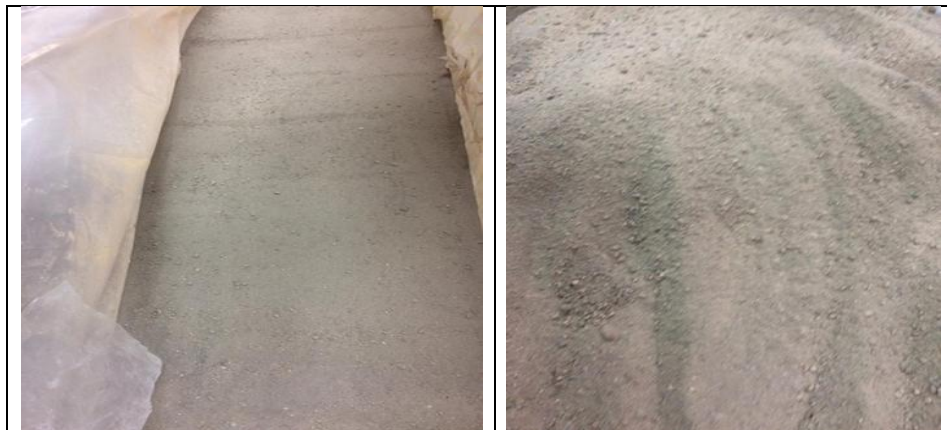
Figure 5. Soil-cement mixture and compacted soil cement.
