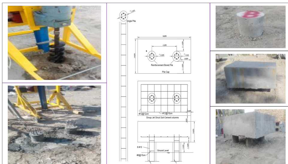
Figure 3. Construction steps of bored pile.
