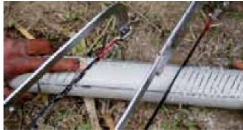
Figure 5. Cutting Slots of PVC Pipes Used In The Well.
