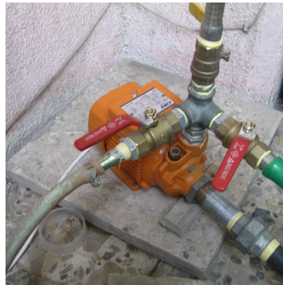
Figure 4. The Centrifugal Pump used and the Relation Between the Head and the Water Flow.
