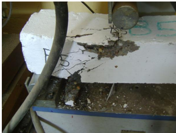
Figure 15. Failure of original B5.
