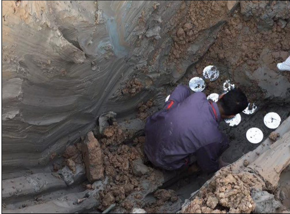
Plate 1. Collecting of undisturbed soil samples from about 3 m deep open bit.
