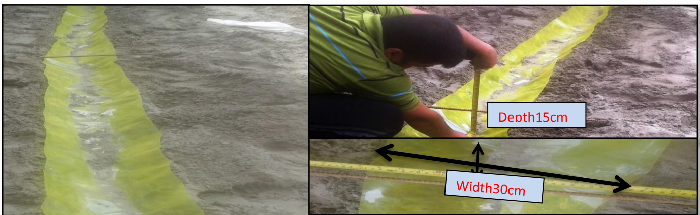
Figure 2. Installation process of the polyethylene sheet below the soil surface.
