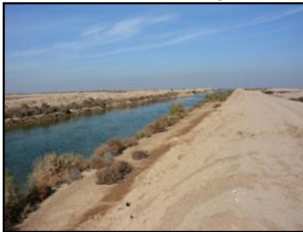
Figure 3. A snapshot showing a general view of inlet canal.
