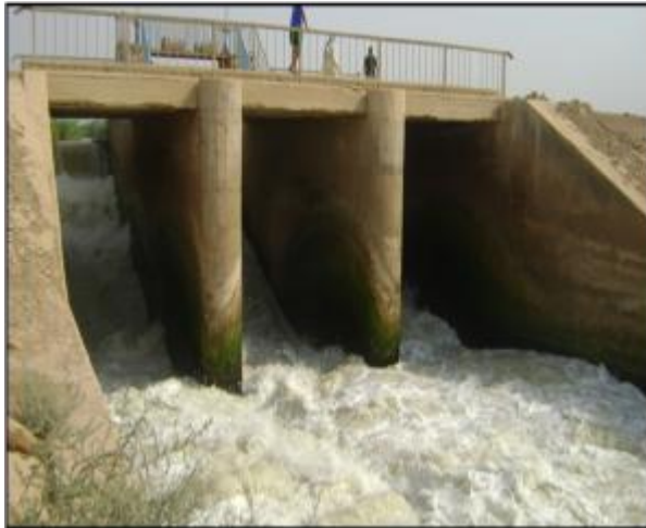
Figure 9. The cross regulator of the bypass canal.
