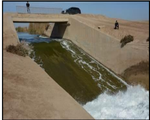
Figure 10. The conjunction structure of the bypass.
