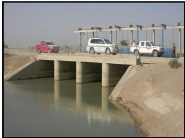
Figure 4. The cross regulator of Addalmage intake canal.
