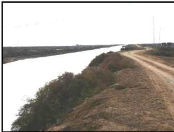
Figure 5. A snapshot showing a general view of escape canal.
